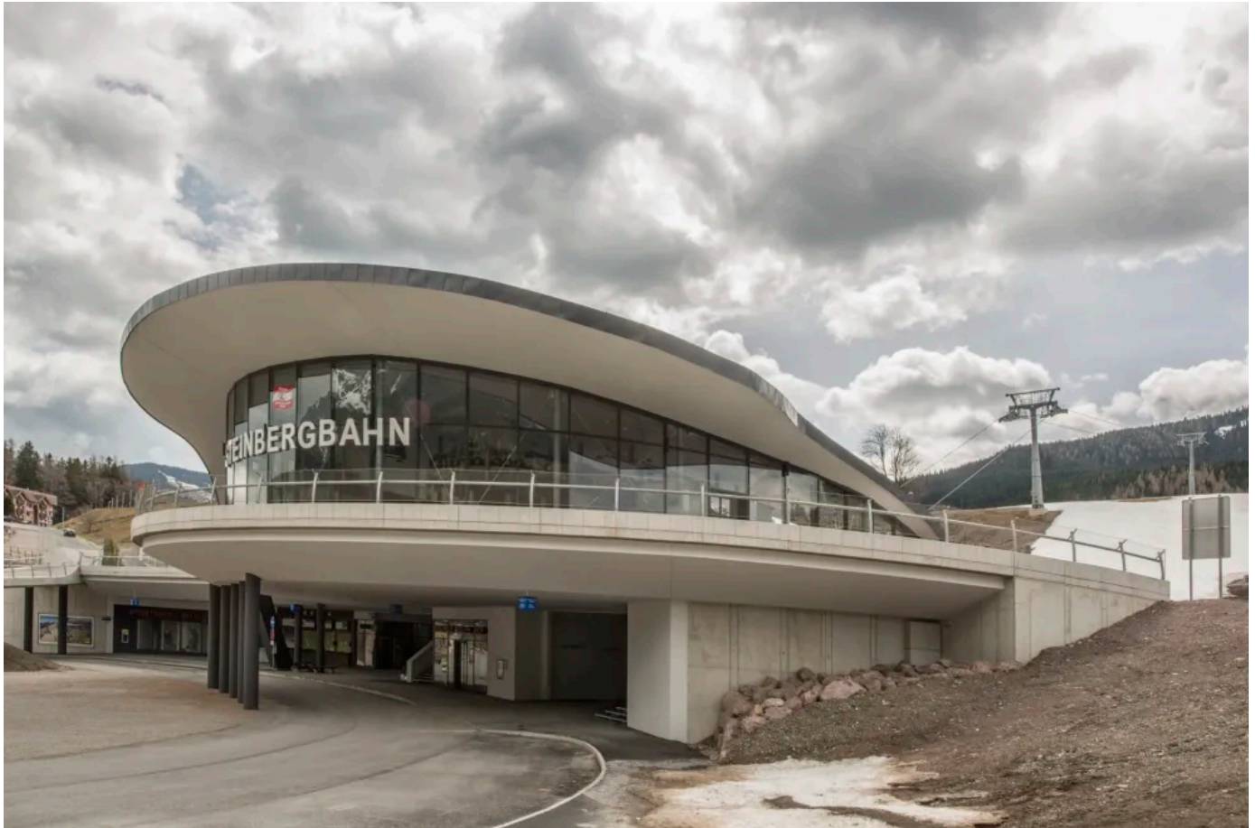
Talstation Steinbergbahn Leogang ©BIRGITPICHLER
