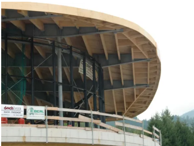
Talstation Steinbergbahn Leogang ©BIRGITPICHLER
