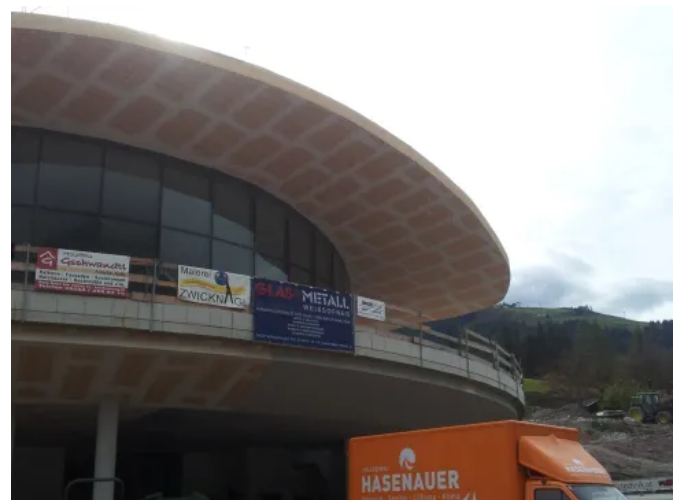
Talstation Steinbergbahn Leogang ©BIRGITPICHLER
