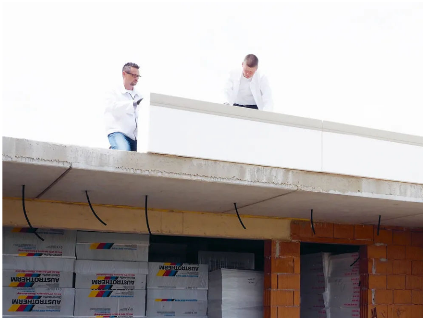
Austrotherm Attikaelement
