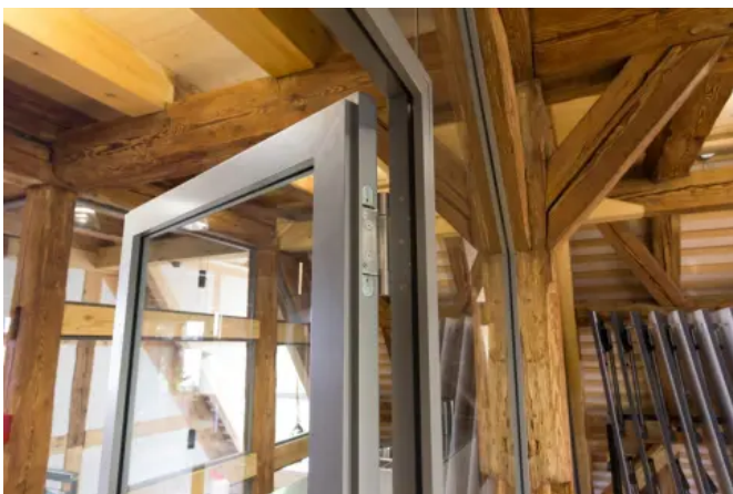
Küffner Aluminium-Rahmentür ART 55, Banddetail
