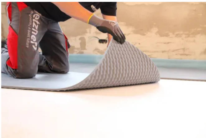
Installation von Acoustic Floor Mat 29
