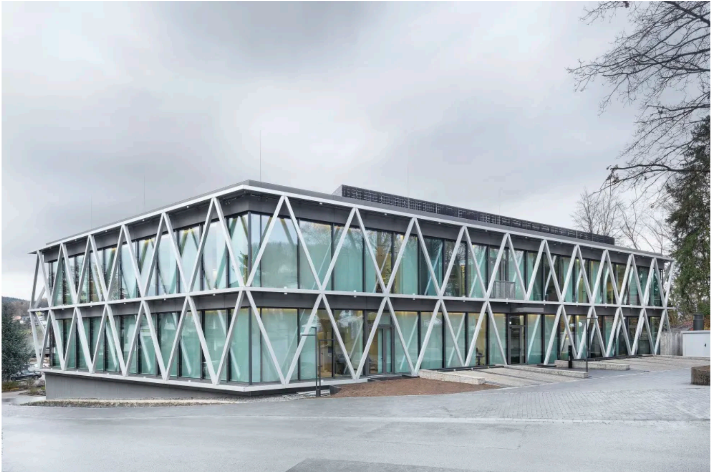
Neubau Balnova, Fertigstellung 2024, Bad Orb; © by diephotodesigbner.de schluchtmann ek (© Ken Achluchtmann)
