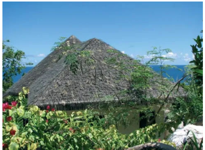
Aluminium "Strohdach"/ Seychellen
