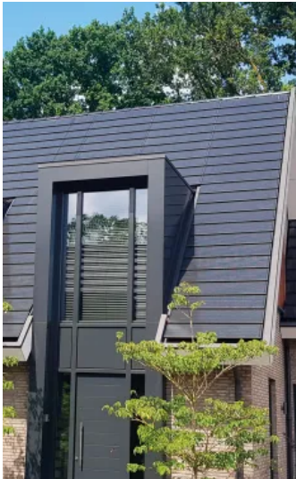
G 10 S PV-Solardach.
