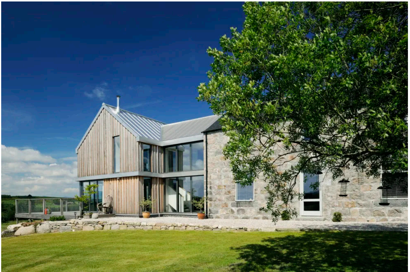
Bogindhu Farmhouse, © Nigel Rigden 2012
