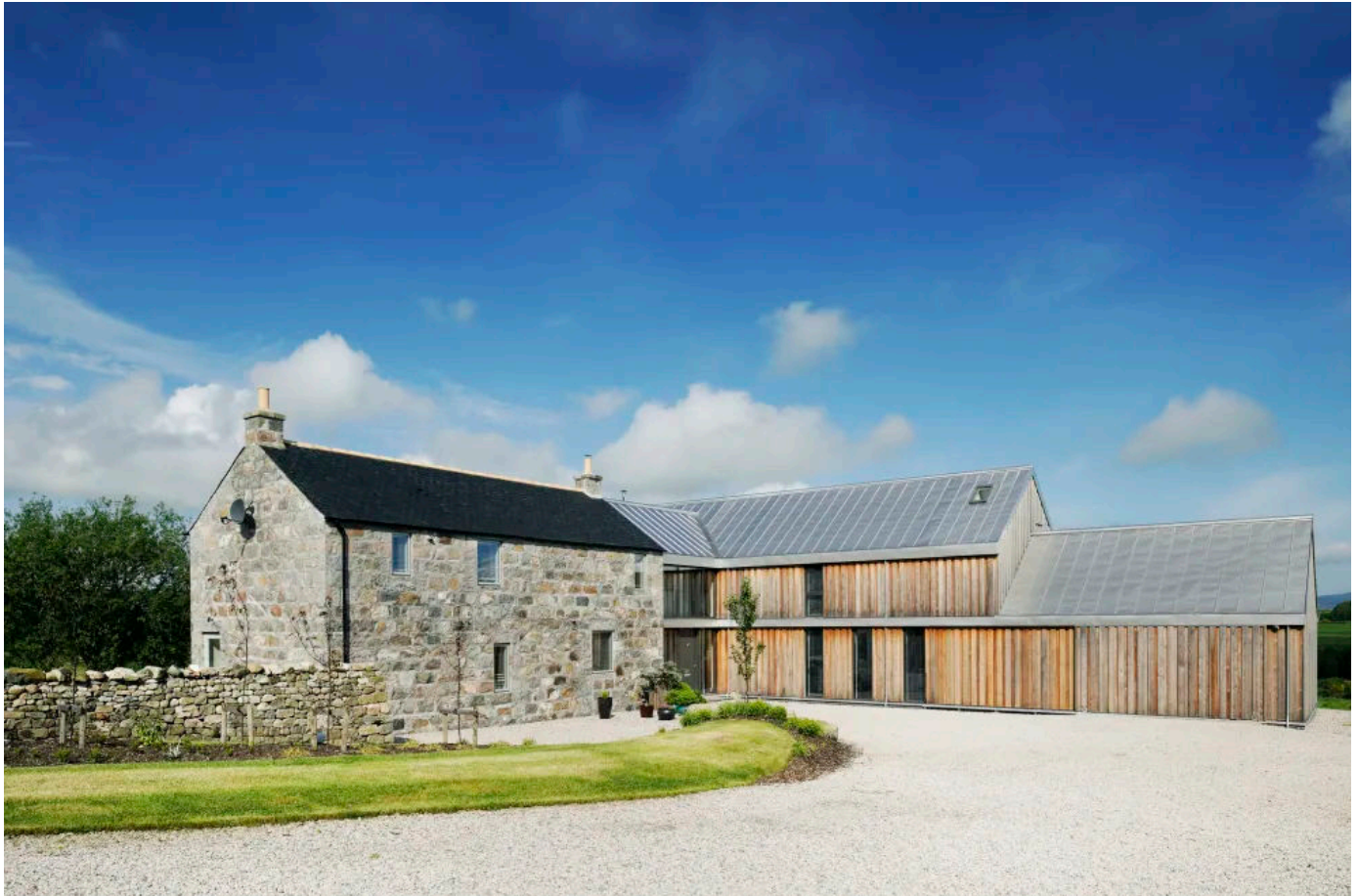
Bogindhu Farmhouse, © Nigel Rigden 2012
