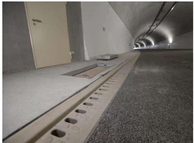
Tunnel Rothenstein - ACO DRAIN® Monoblock T 275 V
