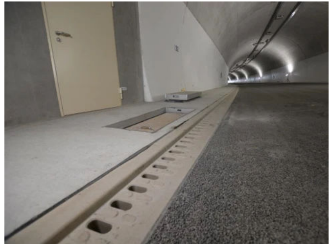
Tunnel Rothenstein - ACO DRAIN® Monoblock T 275 V
