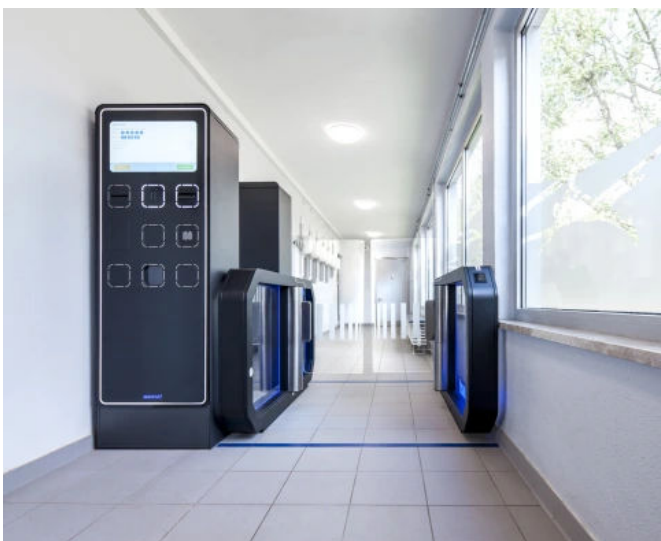
Hallenbad Weissenfels, © André Becker • Photography
