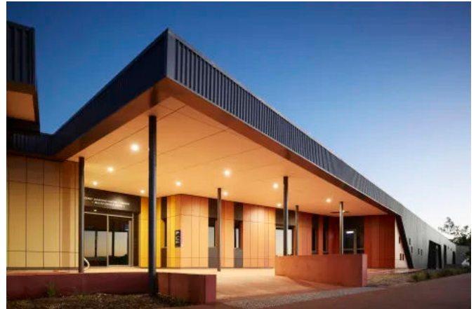
Wickham Community Hub – Wickham, Australia
