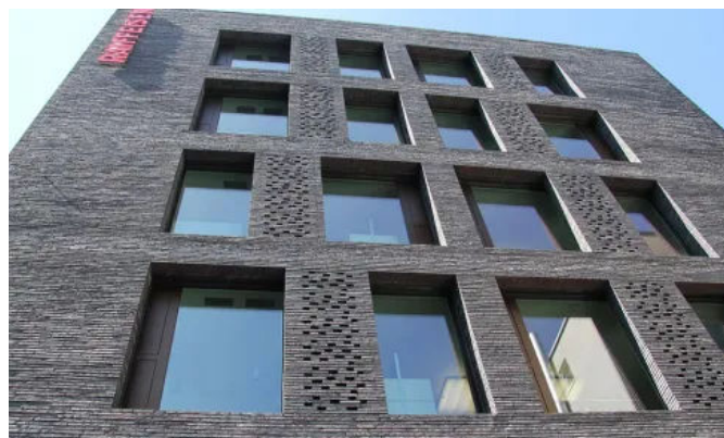
ARGE Raiffeisen St. Gallen
