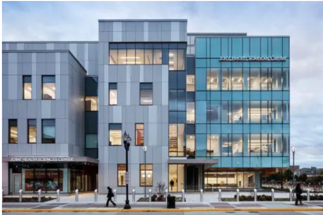
Rowan Joint Health Science Center - Camden, NJ
