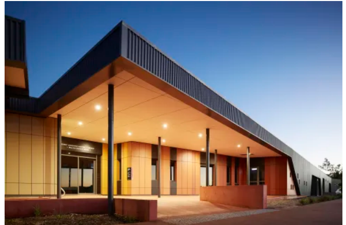
Wickham Community Hub – Wickham, Australia
