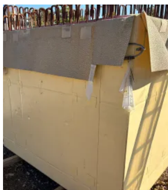
KRASO FBV-Pumpensumpf - Beton
