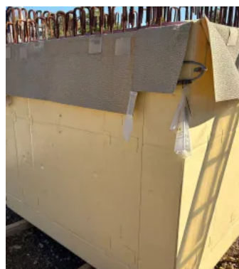
KRASO FBV-Pumpensumpf - Beton
