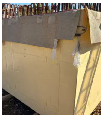
KRASO FBV-Pumpensumpf - Beton
