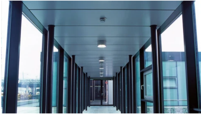
Metall-Flurdecken Armstrong METAL F-Clip Access, F-H 600, F-H 600 Swing, F-H 600 Swing E130, F-L 601 (© Elisabeth Grebe)
