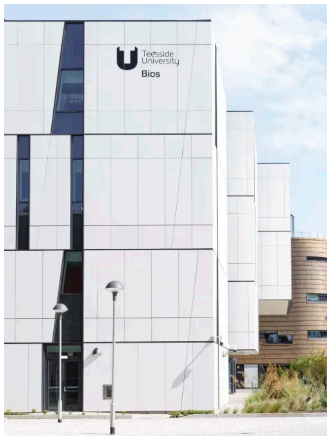
concrete skin Fassadenplatten in BIOS, Teesside University
