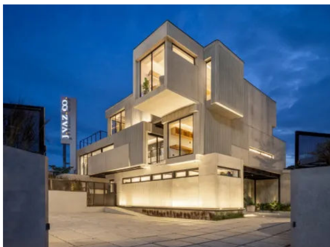
JVAZCO Headquarter Malina
