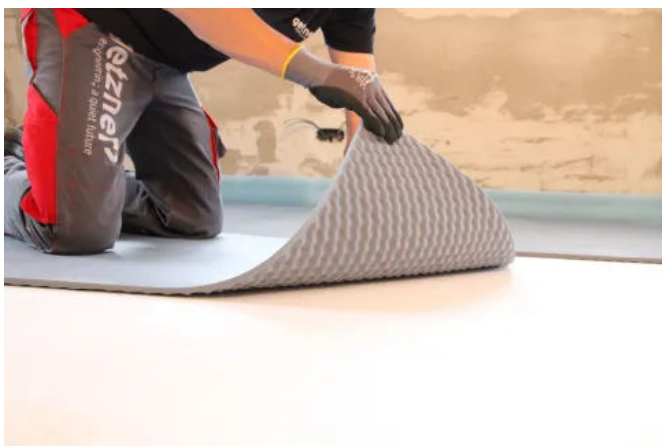
Installation von Acoustic Floor Mat 29
