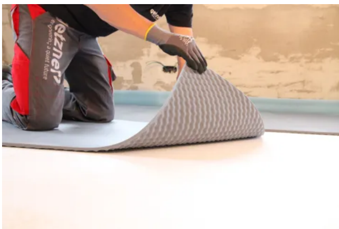
Installation von Acoustic Floor Mat 29
