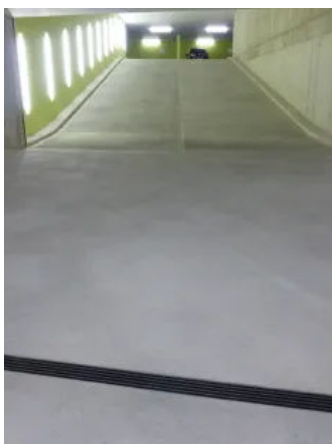
AquaStop in Betonboden
