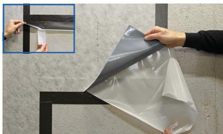
**7** In order to be able to use leftover pieces of the BLANKE DISK sealing film on the surface, the BLANKE DISK TAPE is to be oriented at angle of 90°, on the fleece-free area, to the existing sealing film. Finally the joint area for both the sealing films must be aligned with an overlap of at least 5 cm on the BLANKE DISK TAPE.
