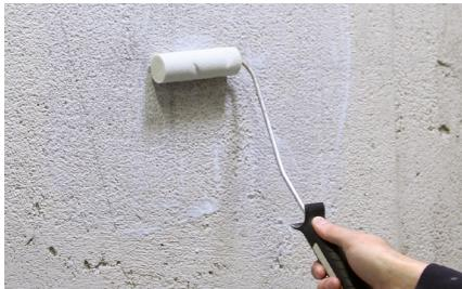
**1** All surfaces must be dry, stable and free of layers that could impair the adhesion. Whereby the evenness must conform to DIN 18202. Depending on their condition wall and floor surfaces must be primed. The manufacturer's specifications on drying times are to be observed.
