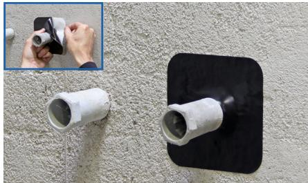
**4** Pipe breakthroughs must also be sealed using BLANKE DISK WM/BM wall and floor sealing collars before applying the sealing film. Care must be taken to have a correct collar for the seal for the pipe extension.
