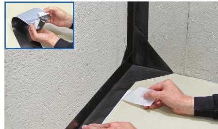
**3** BLANKE DISKTAPE is to be used on all horizontal and vertical corners. Pull up about 5 cm of the parted covering foil, place the corner sealing tape on the surface and, while pull off the foil on the rear-side, press down the film, by hand, bubble free. Repeat the process
