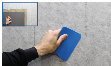
**9** After the compound seal has been created, press on the BLANKE DISK, to create an optimal adhesion to the surface for all components, using the BLANKE DISK Tool pressing aid provided. Finally, without a waiting period, the tile or natural stone covering can be laid using the thin bed method.
