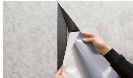
**6** Additional sealing strips are always placed on the fleece-free areas of the BLANKE DISK sealing film and pressed down, bubble free, by hand.
