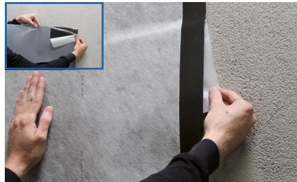
**5** The surface is sealed using BLANKE DISK sealing film. On the rear-side pull off the covering foil about 5 cm at the narrow part, place the film on the surface and by pulling off the rear foil from the covering film step by step press the film bubble free onto the surface by hand.
