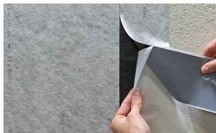
**8** As a last component, the BLANKE DISK AB edging tape is applied to the remaining fleece-free overlapping areas of the sealing film. Here, the covering foil is to be lifted about 5 cm, the edging tape is positioned and, while pulling off the rear foil, is pressed down, bubble free, by hand.
